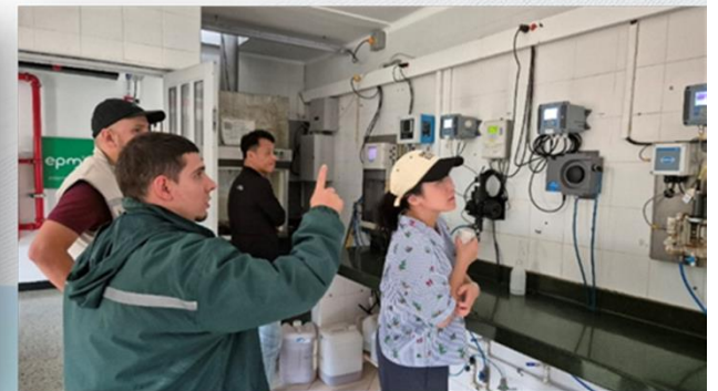
Water Treatment Plant Site Survey
