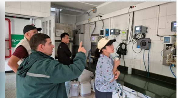
Water Treatment Plant Site Survey
